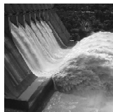
(A) Nagarjuna Sagar dam
